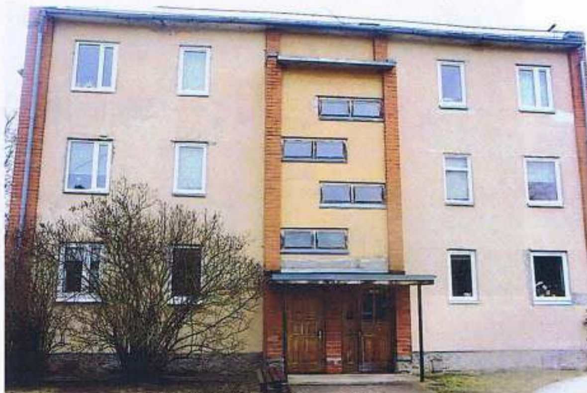
F-8; Ēkas (A) fasādes fragments. A bloks
